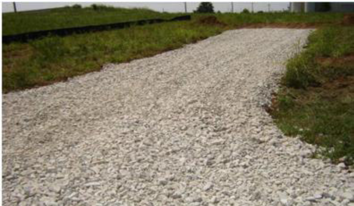
Plate 5: Temporary access track
