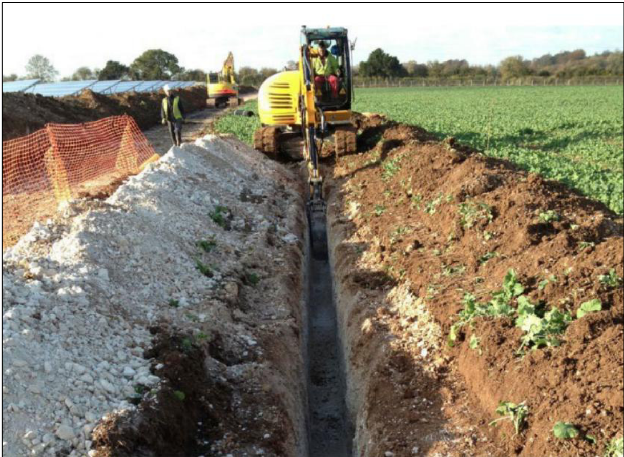
Plate 3: Cable trenching, showing topsoil stripped and set to one side, with subsoil placed on the other side ready for reinstatement (image courtesy of British Solar Renewables)
